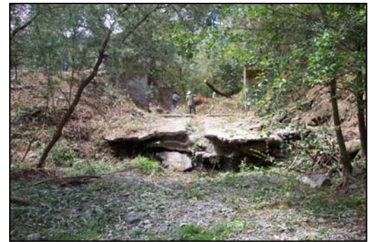
Dam concrete apron in Heath Canyon Creek prior to removal.
