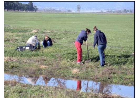
Installing a grass swale on the Klug property. The swale will act as a biofilter and small wetland.
